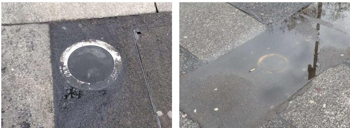
*Up lighters installed with poor drainage*
